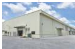
Industrial & Warehouse Sheds
